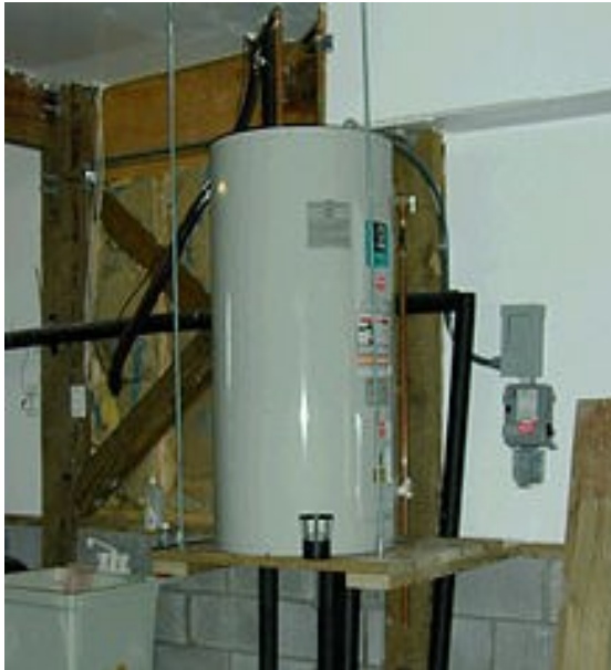
Figure 6.5 Electric tank-type storage water heater
