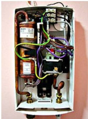
Figure 6.7 Tankless heater circuit
