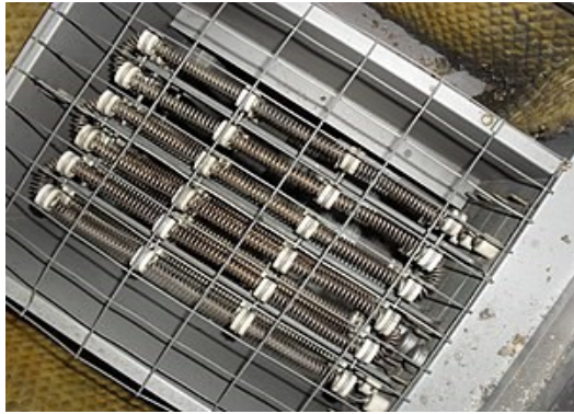
Figure 6.1 30 kW resistance heating coils
