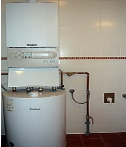
Figure 6.6 Gas furnace (top) and storage water heater (bottom)
