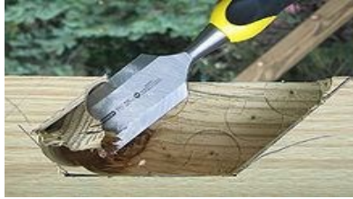
Figure 2.11 A sharp wood chisel in combination with a forstner wood drill bit is used to form this mortise for a half-lap joint in a timber frame.
