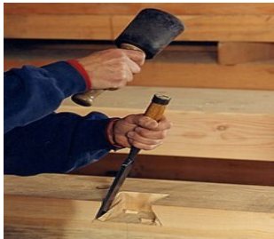
Figure 2.12 A worker uses a chisel to put the finishing touches on a dovetail joint for a timber frame.
