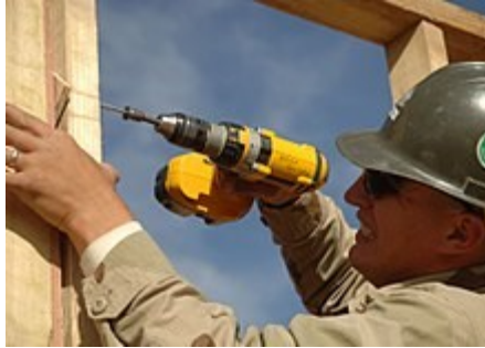
Figure 2.7 Driving a screw with a cordless drill
